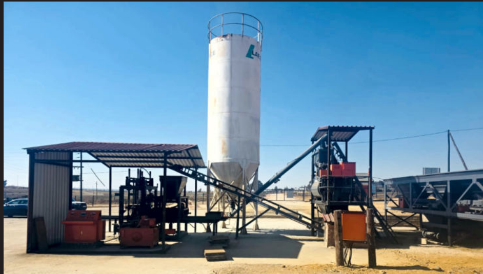
The eMakhazeni Brick Manufacturing Plant in Siyathuthuka, Belfast, is producing approximately 4 000 bricks per day ahead of its official opening on 27 October 2026.
