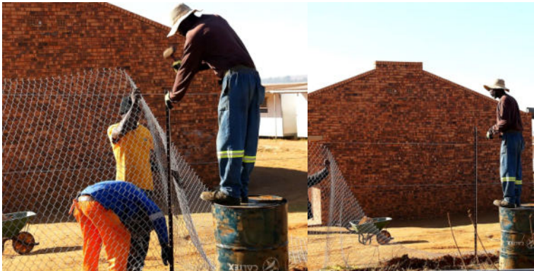
Strengthening school safety through the construction of a new perimeter fence at Mafa Max Motloung Secondary School
