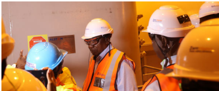
President Cyril Ramaphosa inside the power-generating plant
